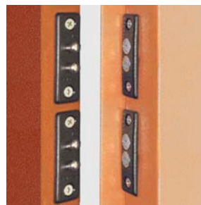
Double electrical contacts between leaf and doorframe
